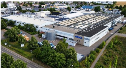
A PVT system supplies the MAHLE plant in Vaihingen an der Enz with solar power and heat, making the plant's heat supply almost entirely independent of fossil fuels.
